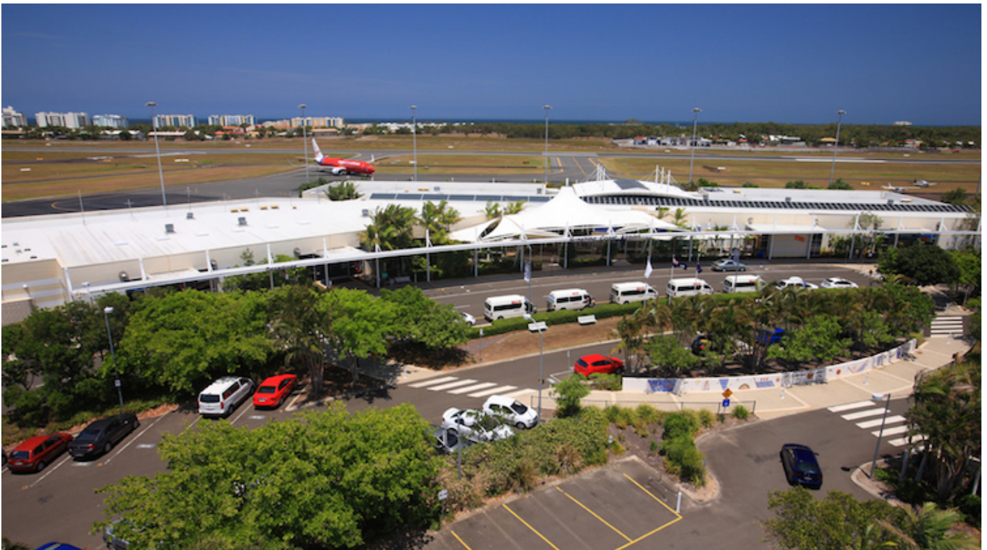
A file image of Sunshine Coast Airport. (Sunshine Coast Airport)
