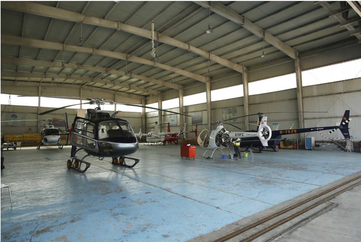
Beijing Capital Helicopter's Hangar and Maintenance Facilities at Beijing's Badaling Airport, the main general aviation airport in the thriving Chinese capital
